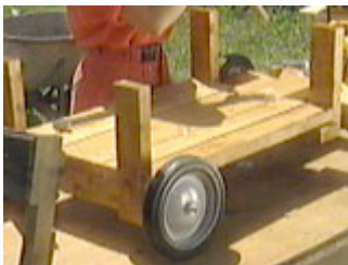
Install a floor and side supports
