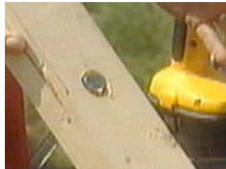
The bolt head should fit below the surface of the 2x4
